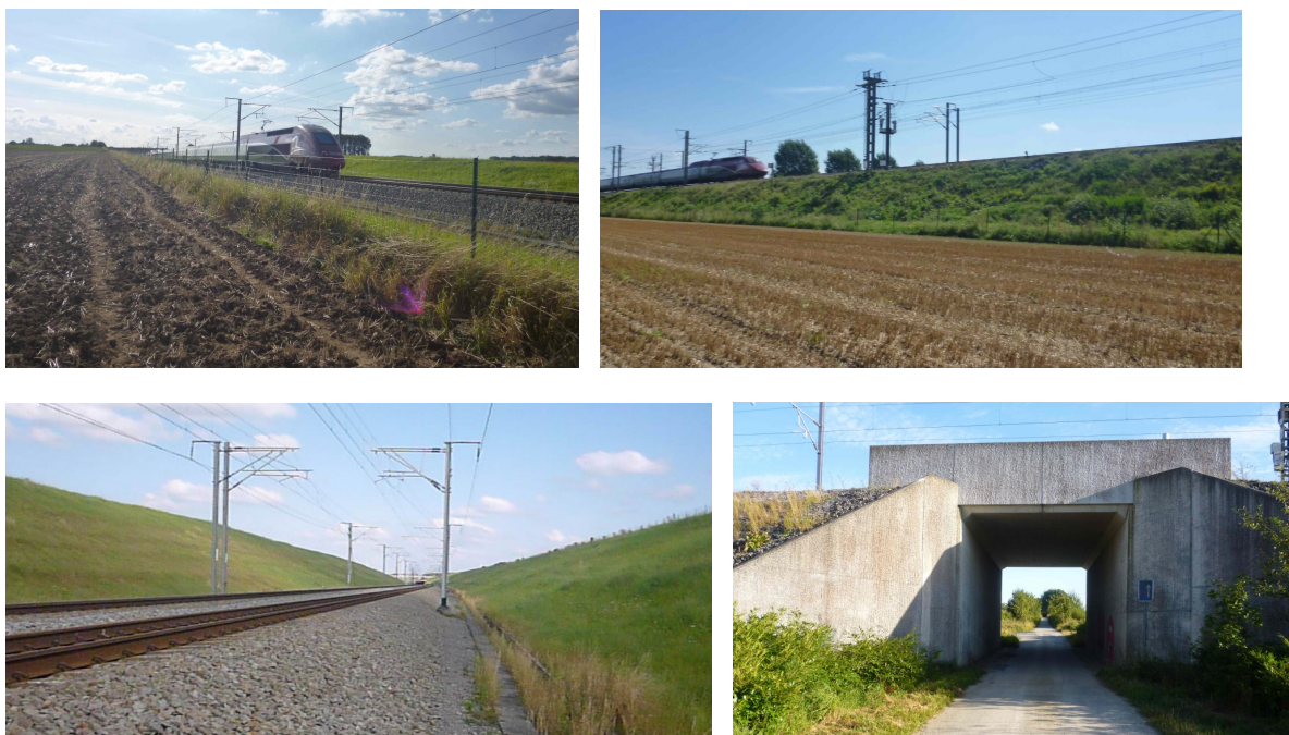
Figure 2 – Top left: site 1 (at-grade). Top right: site 2 (embankment), Bottom left: site 3 (cutting), Bottom right: site 2 (abutment)
